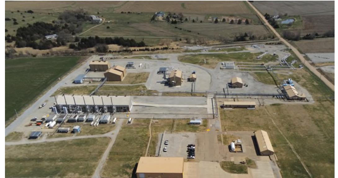
Compressor Station in Beatrice, Nebraska
