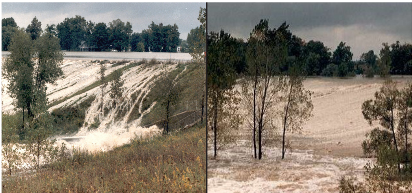
Figure 4: Examples of Dam Overtopping During a Flood
