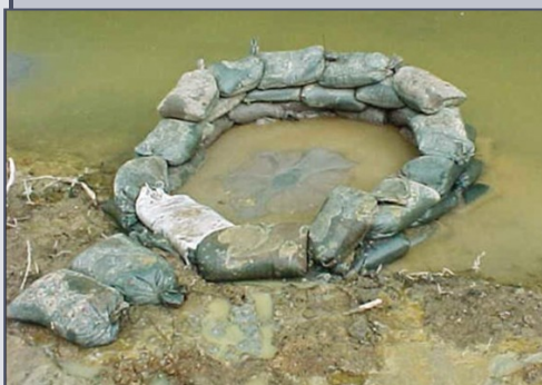
Sandbags surrounding a boil on the downstream side of a dam to pond water and create back pressure. (Photo source: USDA)
