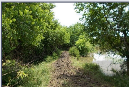
Trees make inspecting the dam difficult and provide attractive habitat for burrowing animals.
