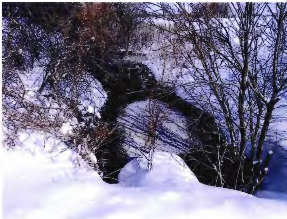
View south of ditch downstream of culvert B
