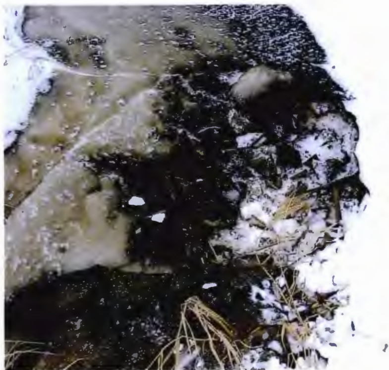
Broken crust of ice at culvert inlet at Stop #4
