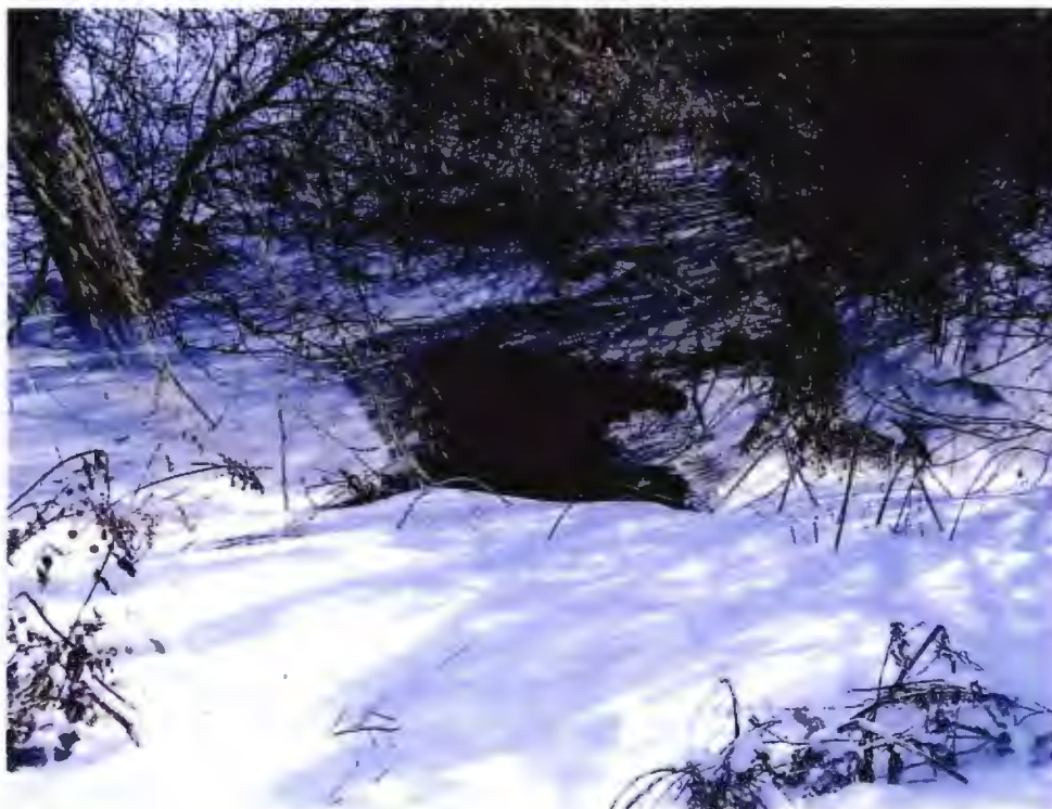
View east of ditch downstream from culvert A
