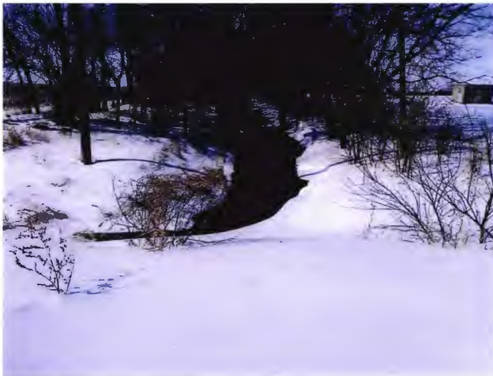
View north of ditch upstream from culvert C
