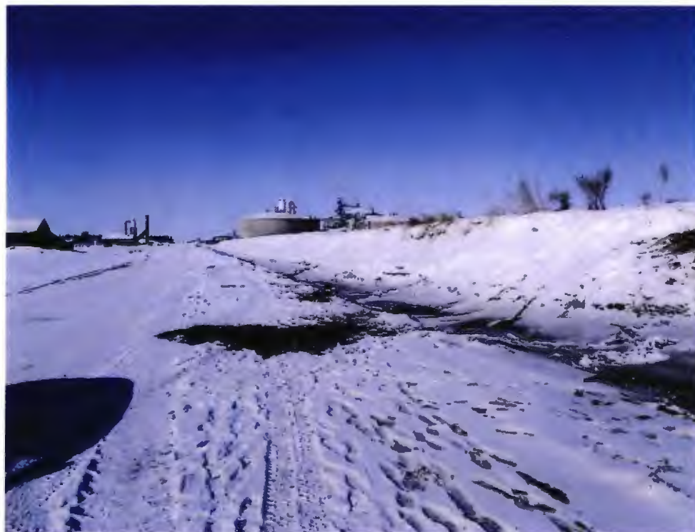
View west of road ditch with digester in background
