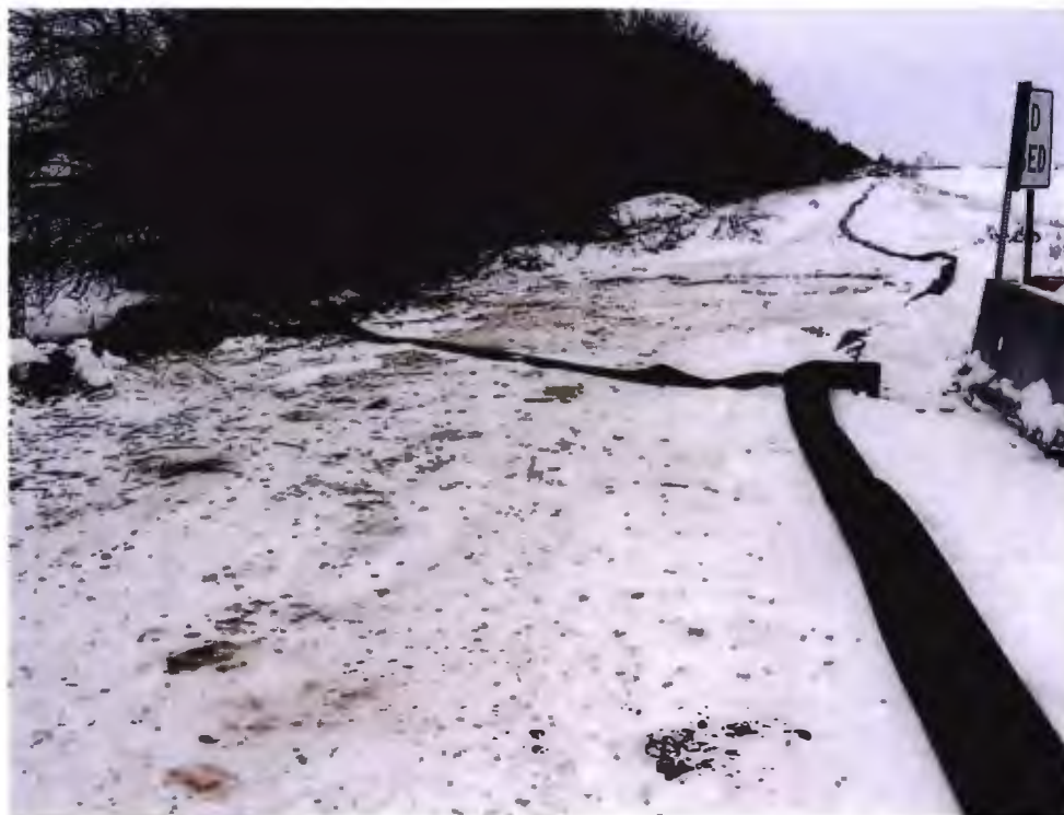
View north of piping laid out at Stop #5
