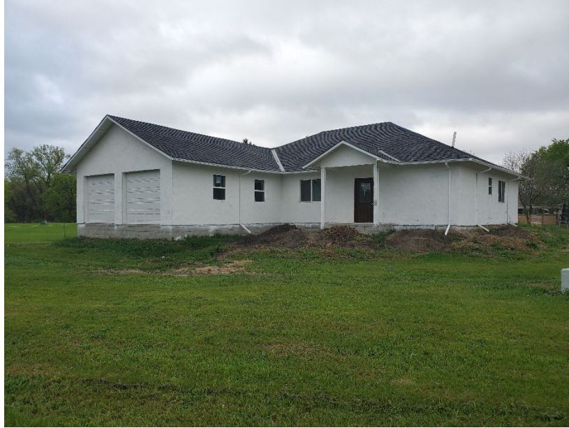
Figure 20: Structure in flood fringe elevated on backfilled block foundation in Schuyler. (DWEE, 2025)
