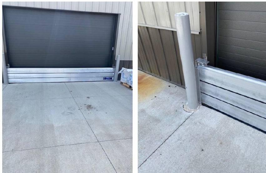
Figure 21: Dry-floodproofing flood shields installed on a large garage in Burt County. (Ann Chytka, 2024)
