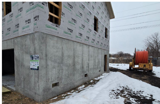
Figure 25: Structure elevated above enclosed foundation under construction in Inglewood. Spaces to later install engineered flood vents can be seen. (DWEE, 2025)
