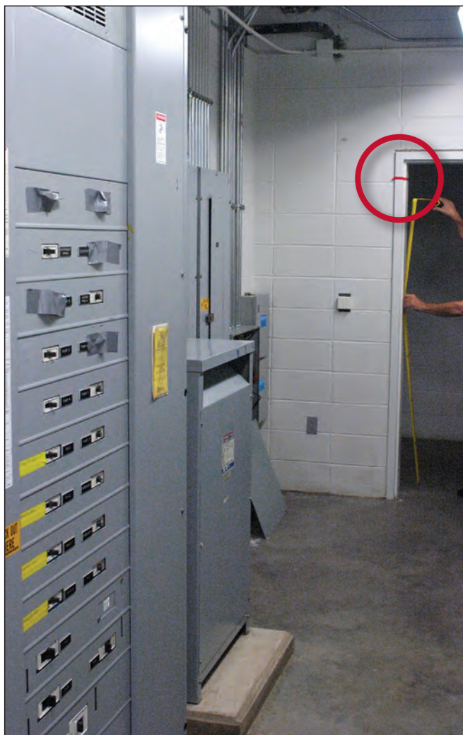
Figure 4-16. Main electrical service switchboard inundated by floodwaters that rose to the red mark on the doorframe (Cedar Rapids, IA, 2008)
