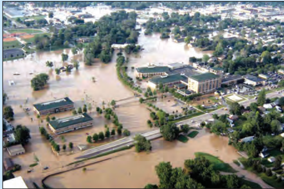
Figure 4-7. Floodwaters surround Columbus Regional Hospital in 2008
