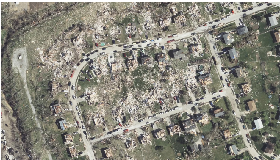
On April 26, 2024, several communities were struck by tornados. Shown here are damaged properties along Old Coach Road and Arabian Road in the Elkhorn neighborhood, that are also within the mapped flood hazard area of West Papillion Creek. Image by Vexcel Imaging.
