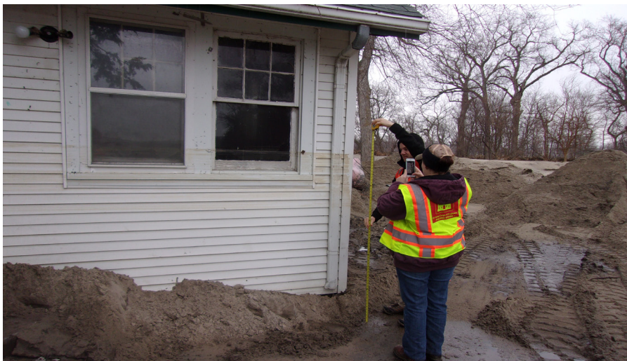
Damage inspection and high-water mark recorded at Waterloo home on March 29, 2019, after historic flooding
