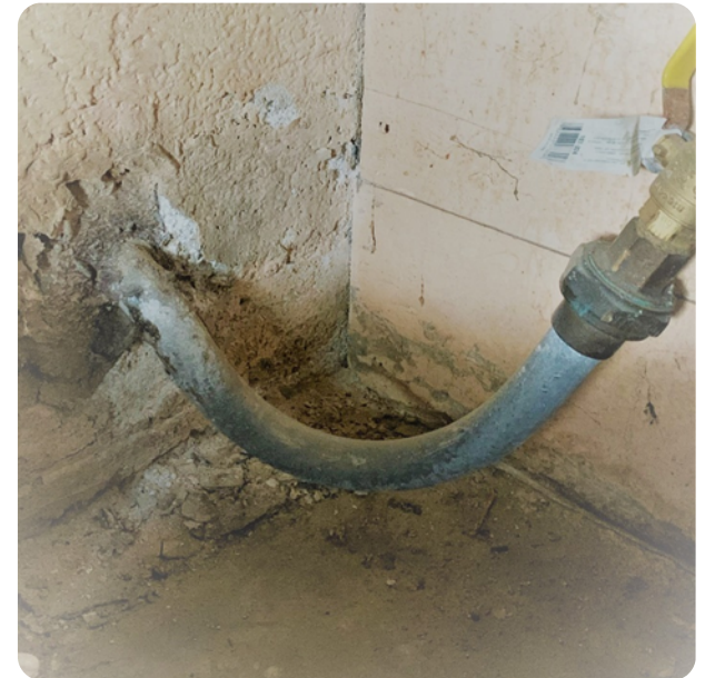
Picture of Lead Service Line in Home in North Platte, NE
