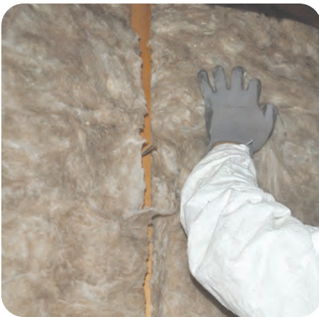
3. Install batts with minimal compression
