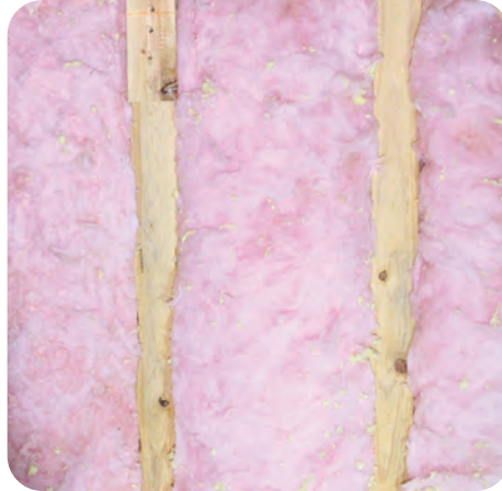
2. Cut batts for exact fit
