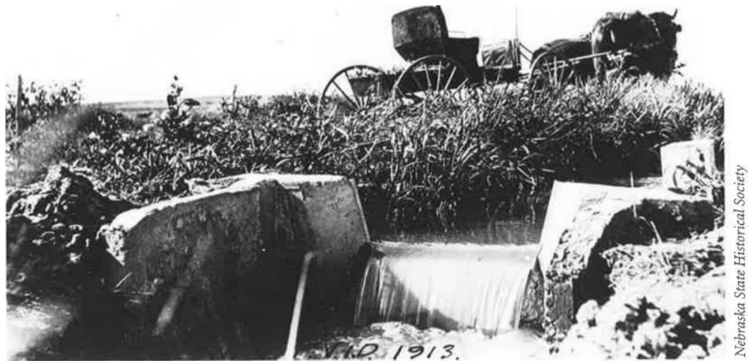
A weir in an irrigation canal, probably in Hitchcock County, 1913.
